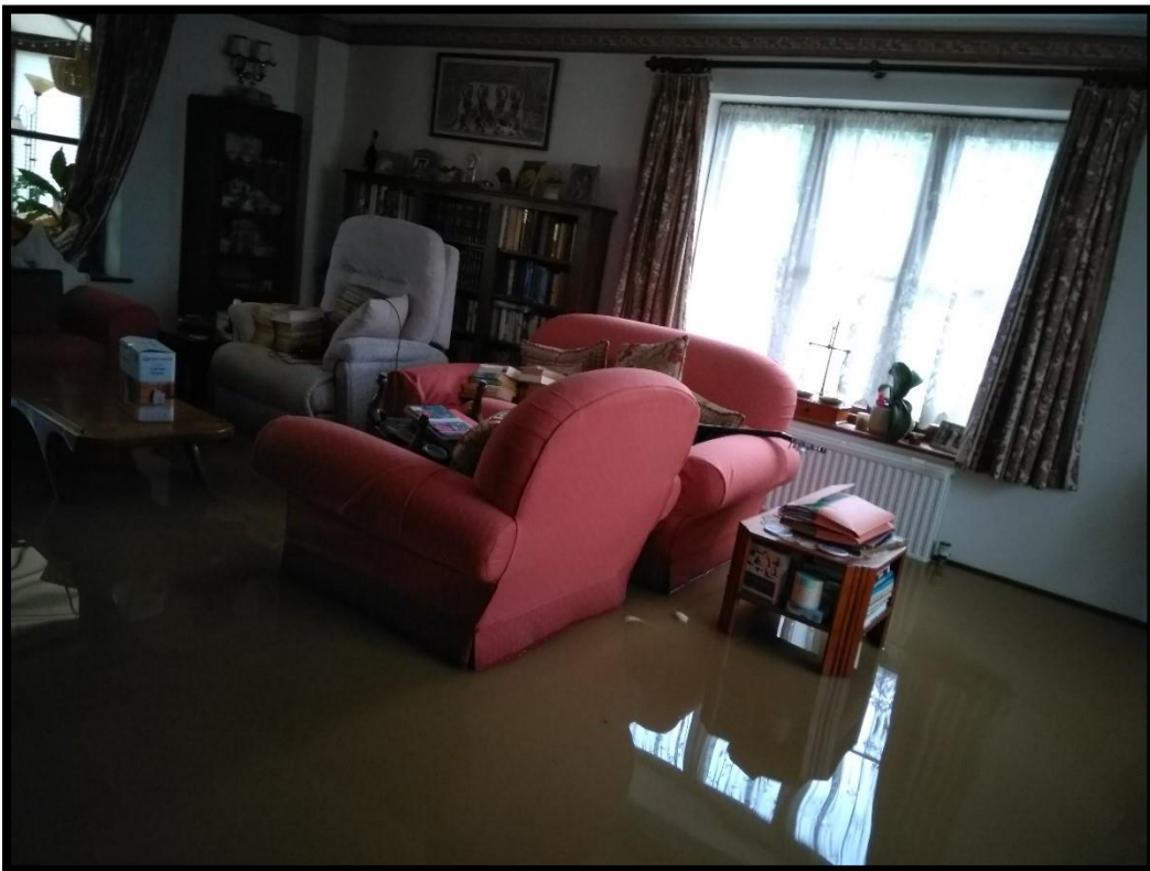
Internal Flooding extents
