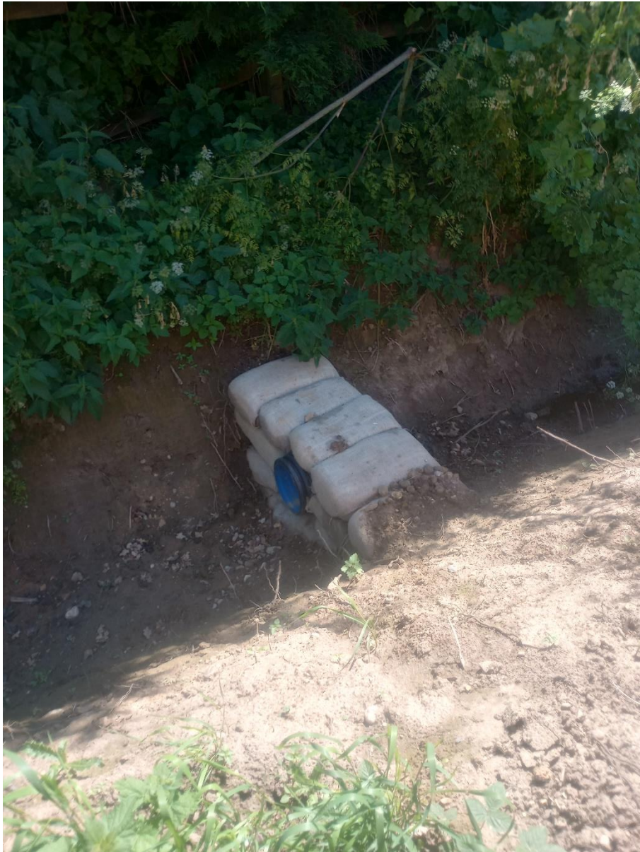
Photo 5 – Installed hessian sandbag headwall in highways ditch line.
