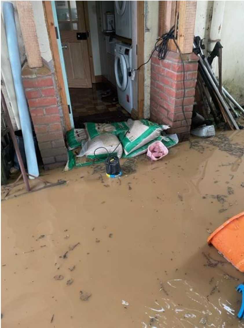
Photo 3 – Internal flooding photograph provided by resident in August 2023.
