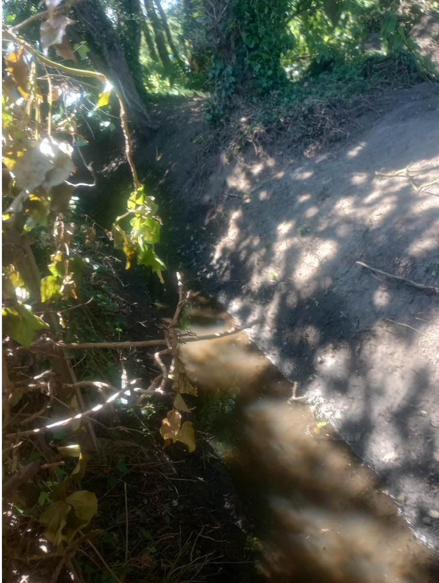
Photo 7 – Private ditch line.
