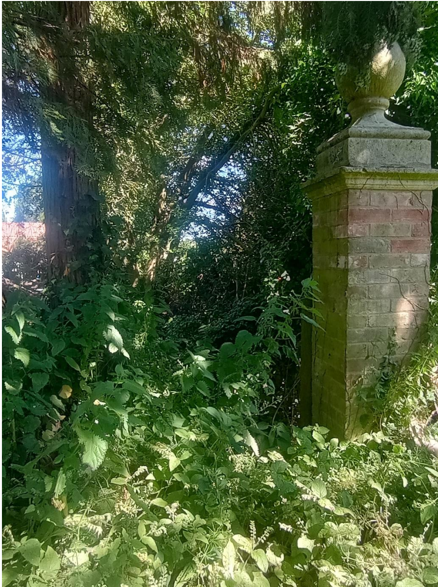
Photo 6 – Access to private ditch line.
