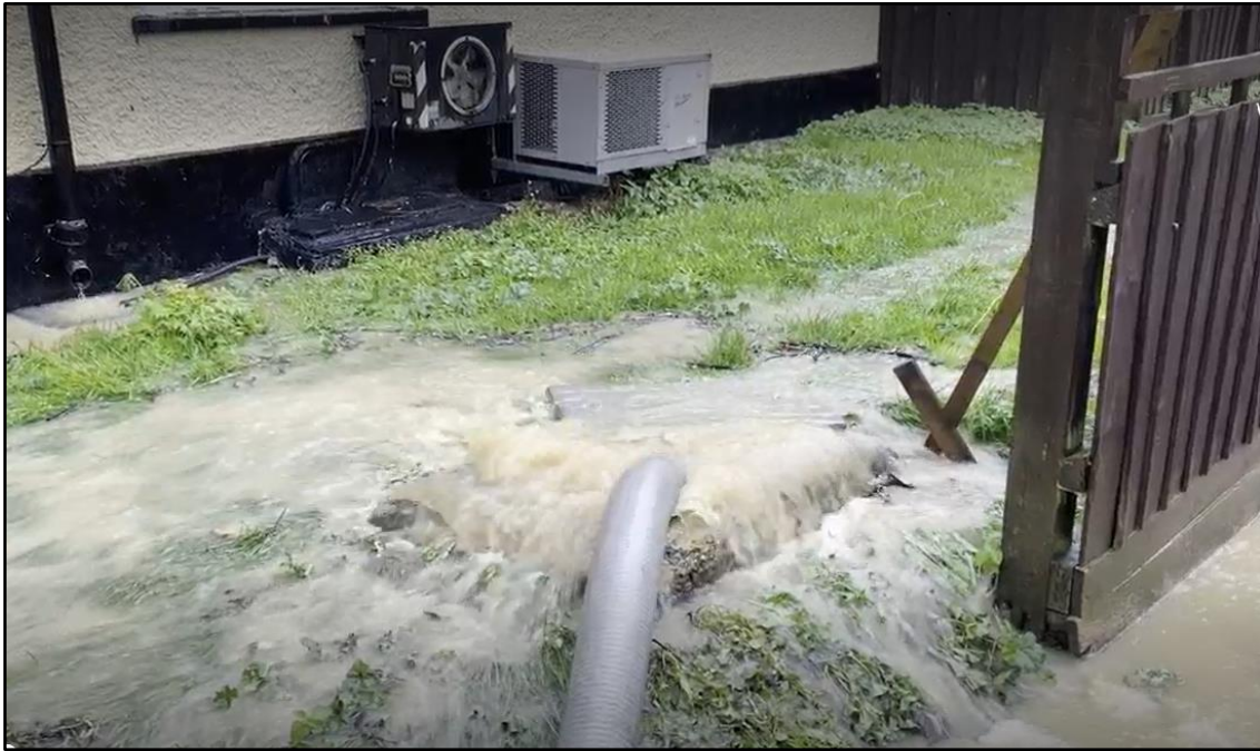
Image 6 - Surcharging manhole outside Barley Mow public house
