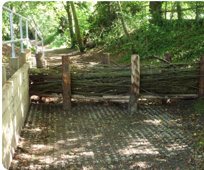
Natural Flood Management – leaky dam.
