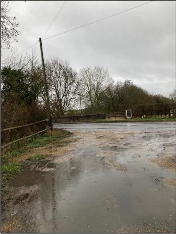
Image 4. Flooding from the highway entering a driveway at the bottom of Swan Hill, A1120 on 21st February 2023, after a couple of hours of light rain
