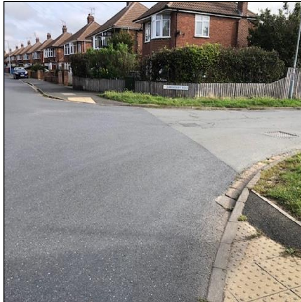
Manholes in Larchcroft Road which were lifted during the flood event
