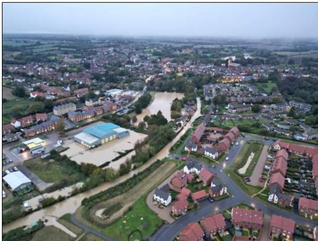
Image 6 - Flooding along Fairfield Road
