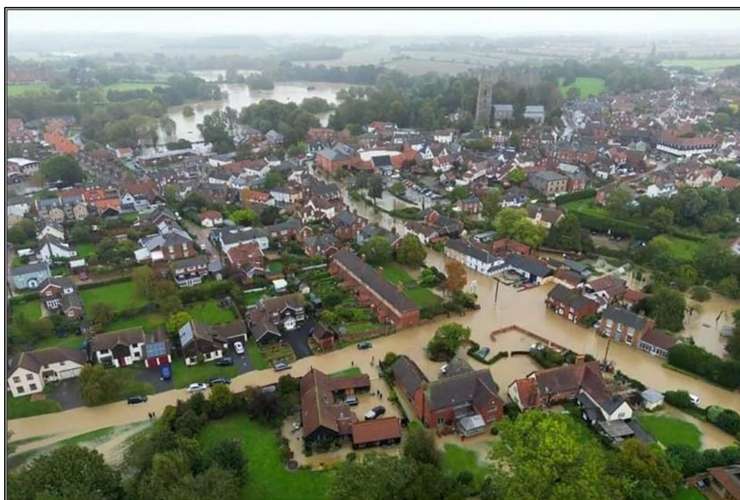
Image 9 - Flooding on Brook Lane and Station Road
