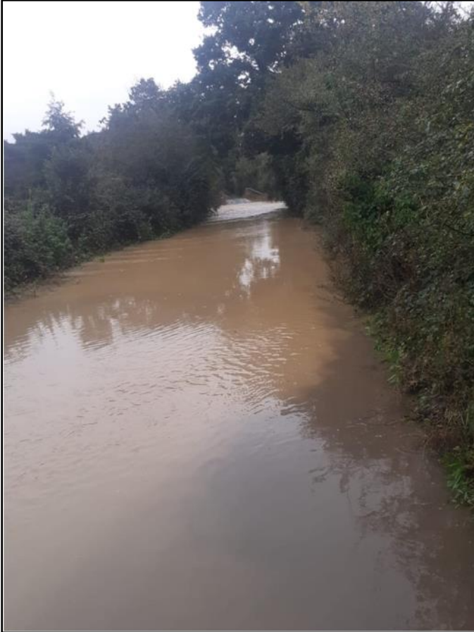
Image 3 Flooding at Boot Street road bridge
