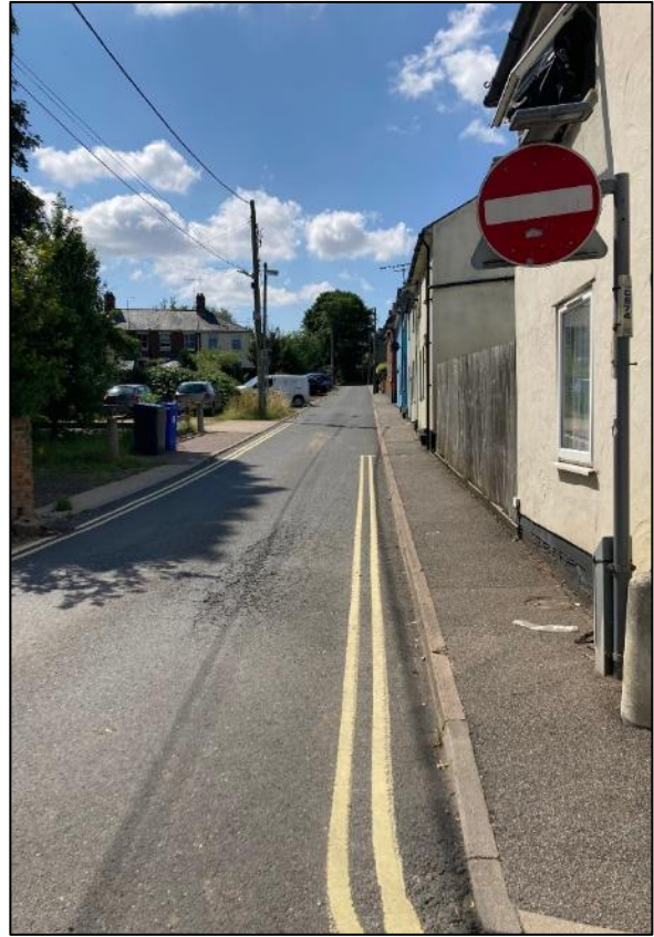
Mill Road, looking upgradient, where surface water travelled down, missing gullies and jumped the kerb into adjacent properties through rear gardens
