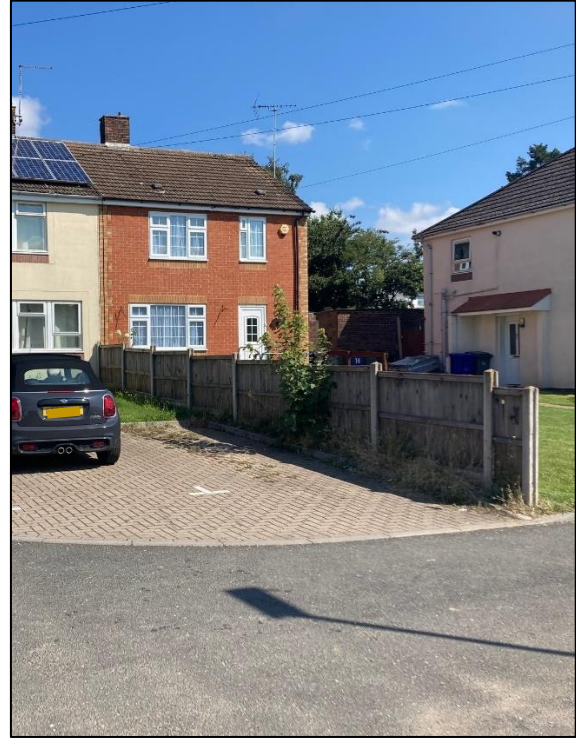
Areas that were previously laid to grass, now paved over to provide parking areas and contributing to runoff
