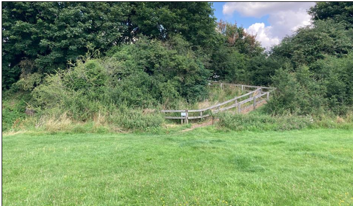
Motts Field (looking north), at point where Stour Brook is culverted under embankment and excess flows combined with surface water overland flows travel eastwards through rear gardens
