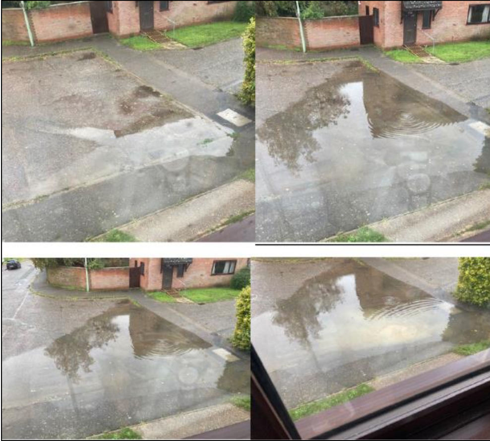
Image 3 - Sequence of flooding from a drainage gully on Pinecroft Way
