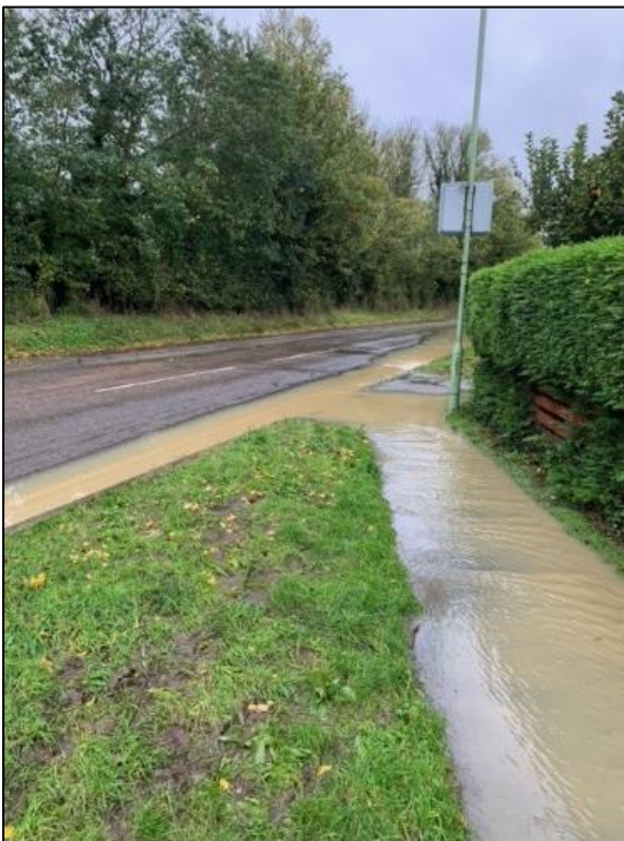
Image 2 - Barking Road floodwater showing flowpath over the dropped kerb
