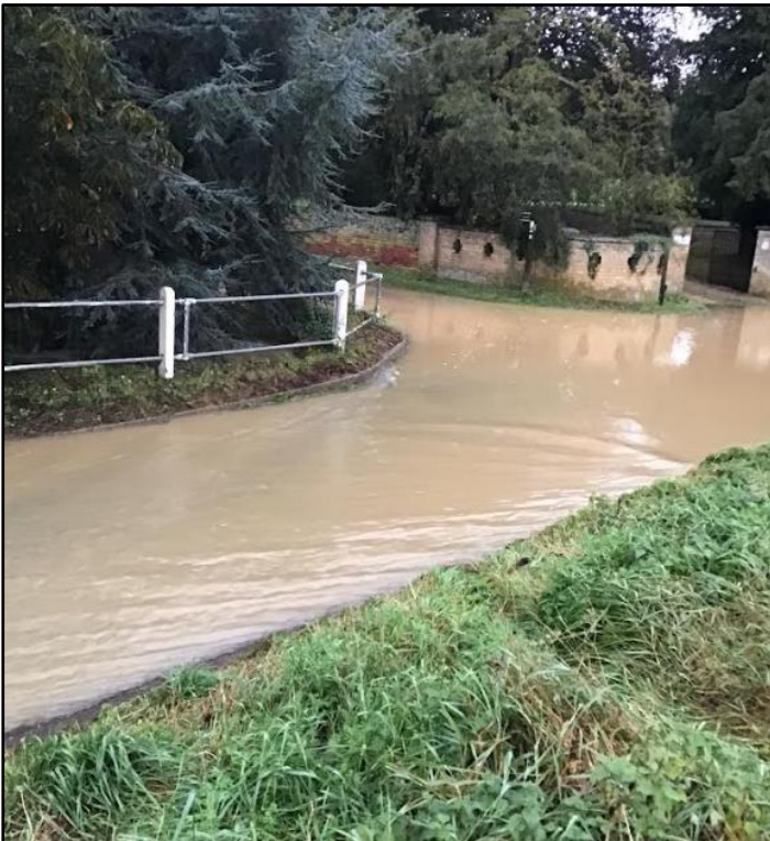
Image 4. Highway flooding outside Brick Lane
