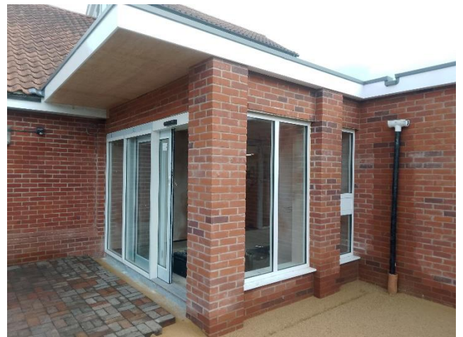
Exterior of new foyer
