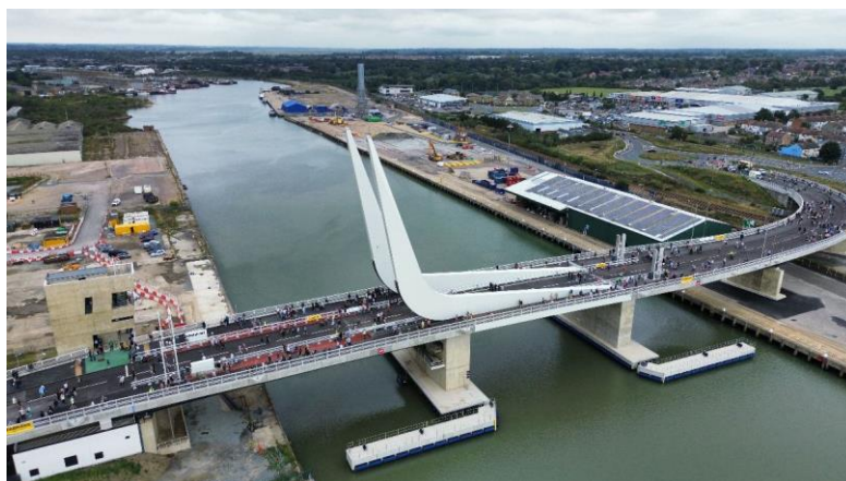
Gull Wing Bridge, Lowestoft
