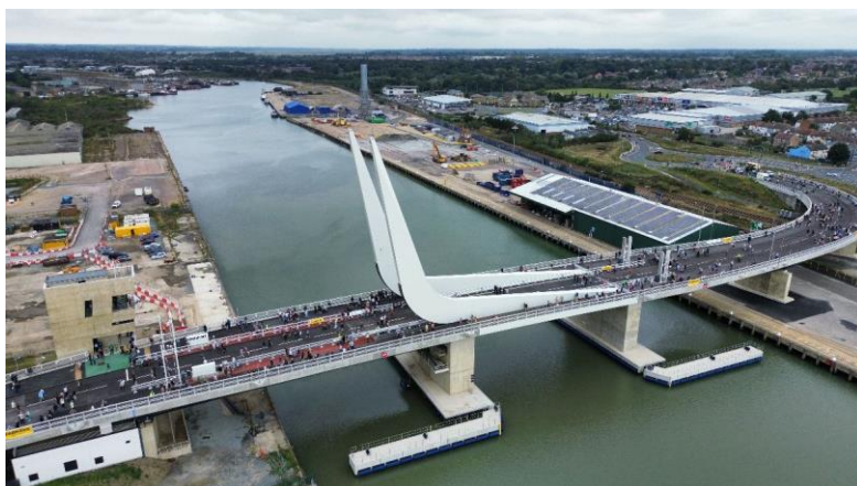
Aerial shot of bridge
