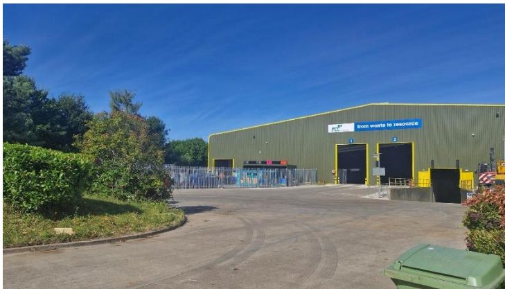
Exterior of new HWRC building
