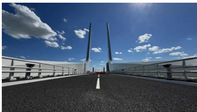
Road surface and bascules
