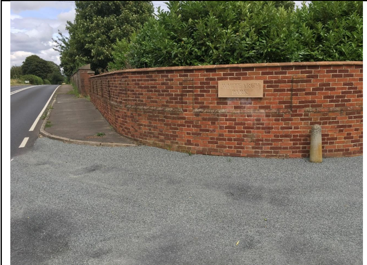
1717_P44_2024 – South footway - Footway surfacing (July 2023)
