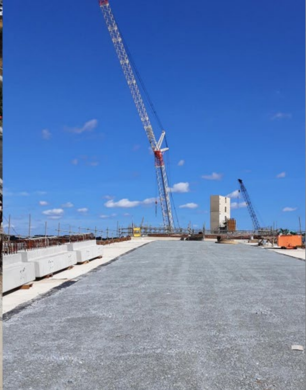
Precast Edge Beam and base course
