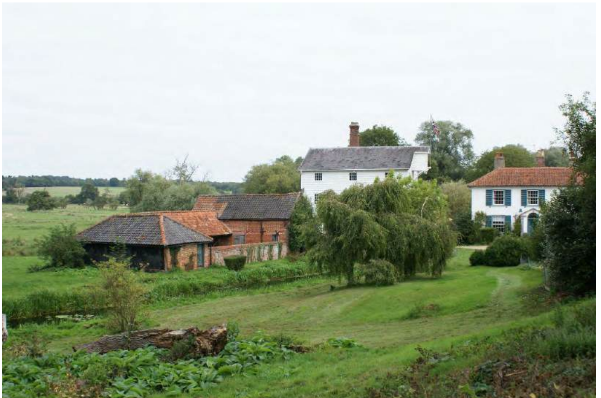
Mill and farm buildings at Low House Farm, Water Mill Lane
